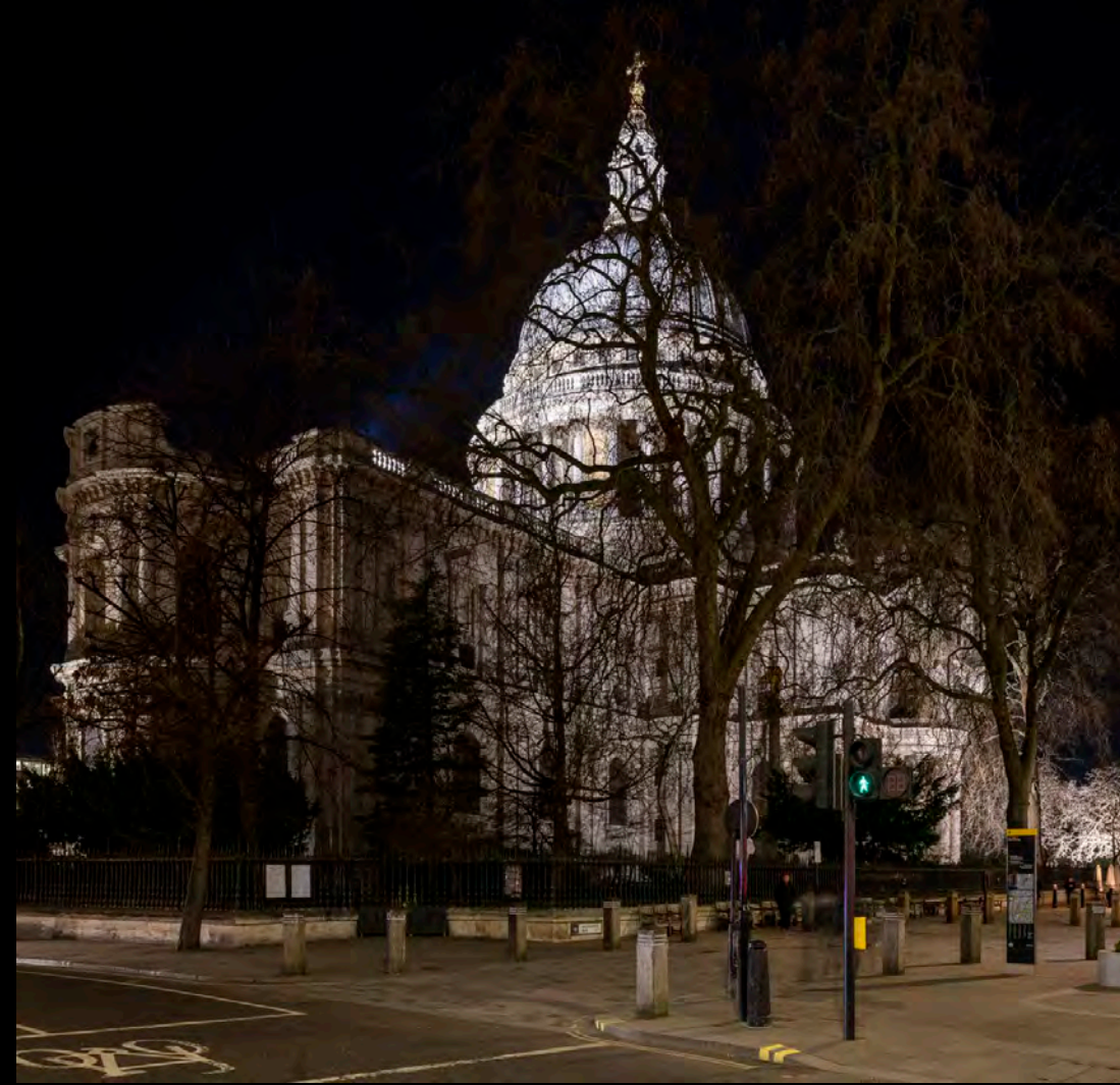
Cheapside – the east end and north facades appear underlit...
