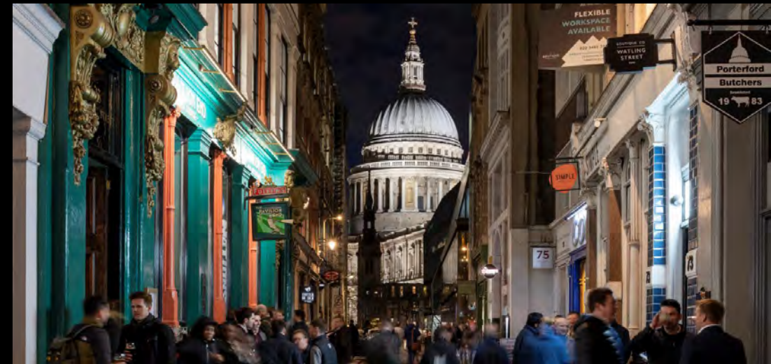
Watling Street – the uneven shadowing of the balustrade to the Stone Gallery is clearly visible...
